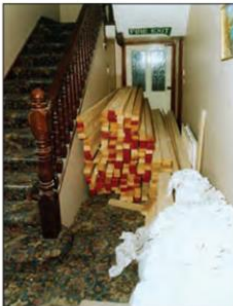
Figure 7.1: A blocked corridor with incorrect signage
