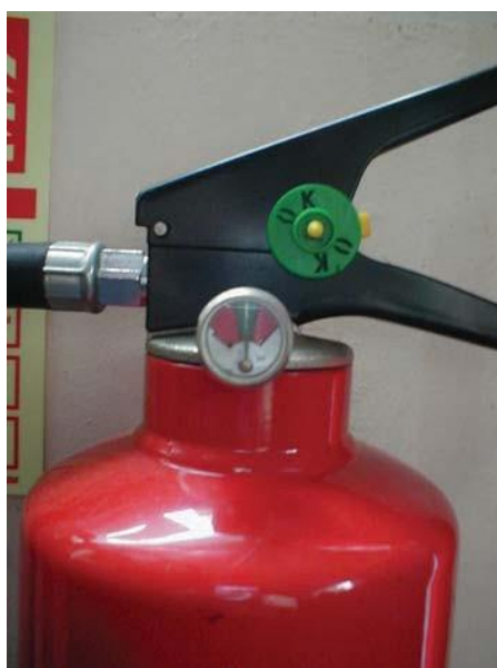
Figure 1.3: Pressure gauge on the neck of a water extinguisher
